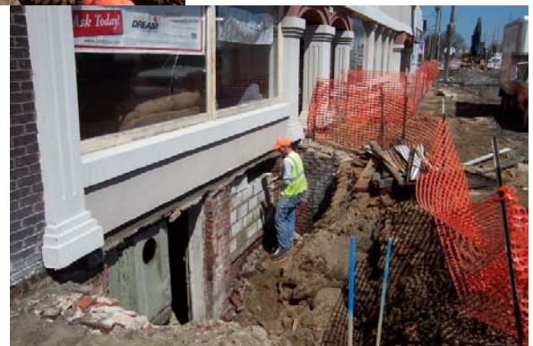
Sealing up the holes before filling this back in.
